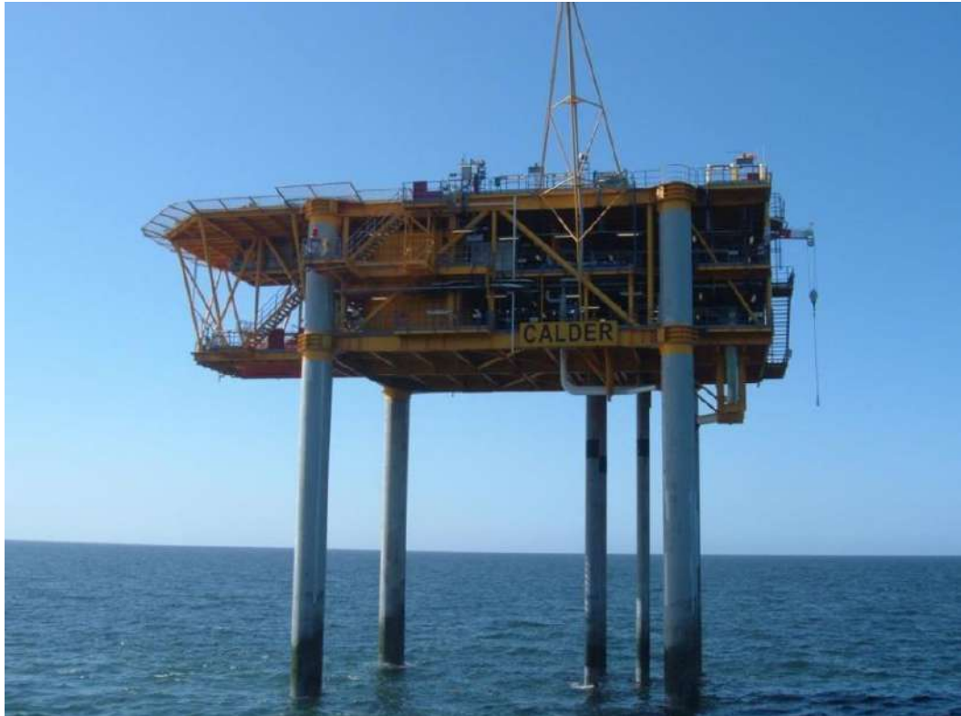
Figure 2.1.4: Photograph of the Calder platform (south face)
