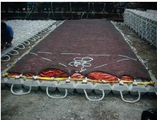
Figure 2.4.18: Typical concrete and concrete froned mattresses (6m x 3m x 0.15m)
